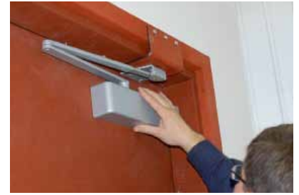
Step 24 - Installing Door Closer Cover
