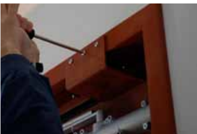
Step 19 - Install Outswinging Door Closer Bracket
