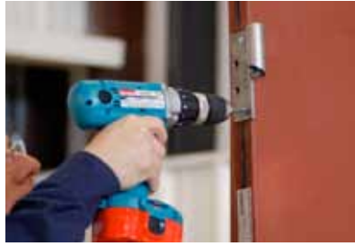
Step 11 - Install Cam Hinge on Door
