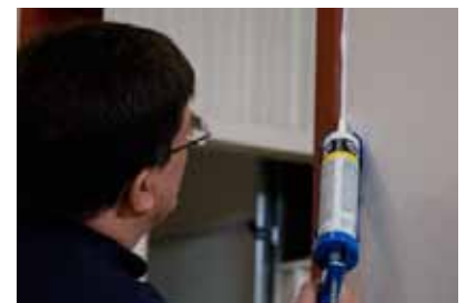
Step 9 - Insulate & Seal Door Frame
