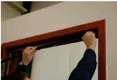
Step 16 - Attaching the Magnetic Seal
