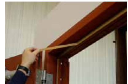
Step 15 - Taping Retainer Cover For Magnetic Seal
