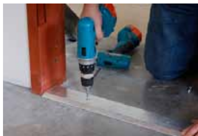
Step 8 - Secure Threshold
