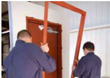
Step 17 - Install Back Frame
