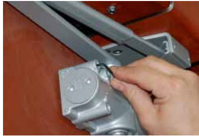
Step 23 - Adjusting the Door Closer
