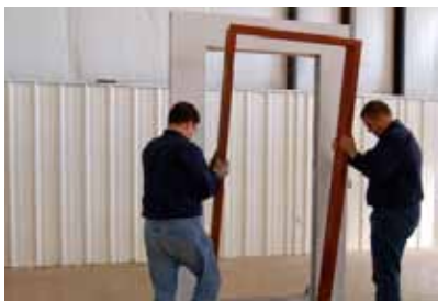
Step 4 - Set Frame in Opening
