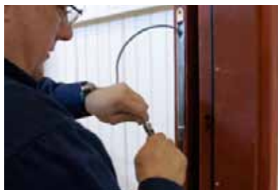
Step 20 - Install EPT to Frame
