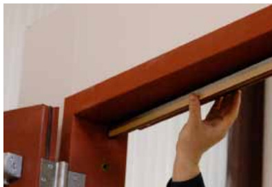
Step 14 - Install Seal Retainer
