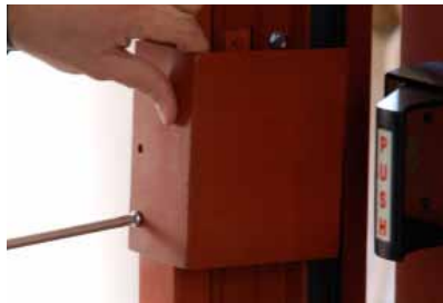
Step 26 - Secure Frame Bracket to the Door Frame
