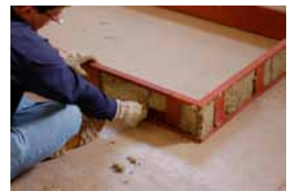
Step 3 - Insulate Frame
