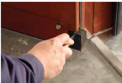
Step 28 - Trimming Seal From Super H Door Bottom
