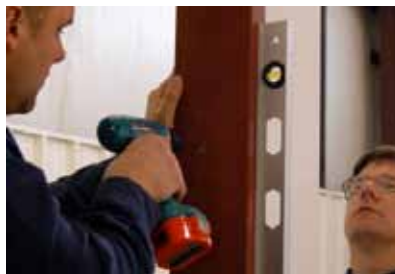
Step 5 - Level & Secure Frame
