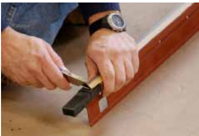
Step 13 - Cut the Seal Retainer to Correct Length
