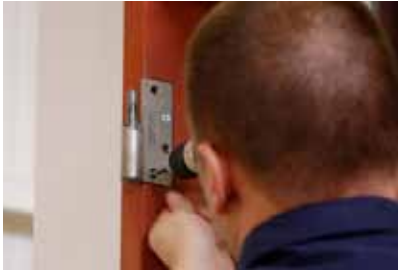
Step 10 - Install Cam Hinge on Frame
