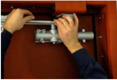
Step 22 - Attaching Closer Arm to Closer
