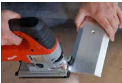
Step 7 - Measure & Cut Threshold
