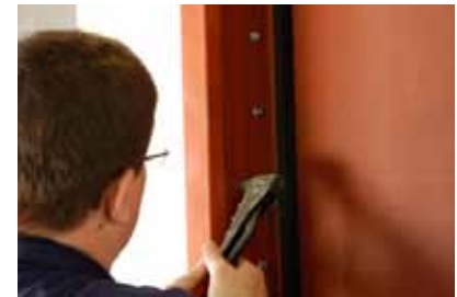
Step 18 - Install Pop Rivets to Secure the Back Frame
